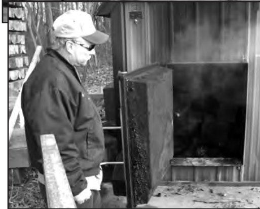
Mill Owner John Falconio opens outdoor furnace which radiant heats sawmill shop floor with sawmill scraps
